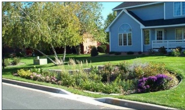
Figure 2. A rain garden installed in the Crystal Lake watershed in Burnsville.
