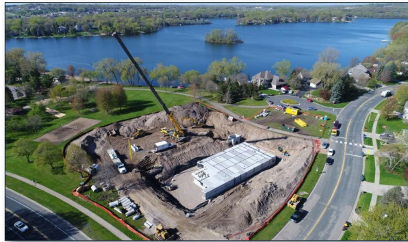
Figure 3. An underground stormwater treatment system reduces contaminated water entering Keller Lake (not visible). Crystal Lake is in the background.
