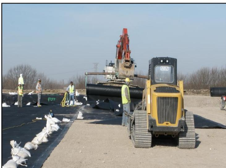
with a spreader bar attachment which remained stationary on the top of the slopes, and a 4-wheeler which pulled the geomembrane into place. Final positioning of the panels was done by hand and included overlapping the panels a minimum of 4 inches to allow for seaming. Photo 4-3 shows the LLDPE line being pulled into place in the non-TSCA dewatering pad.
