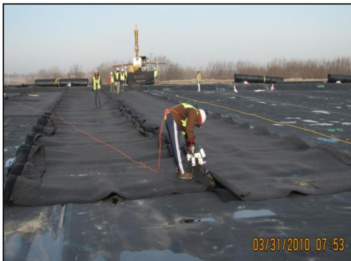
**Photo 4-5. Sewing Geocomposite Layer**
