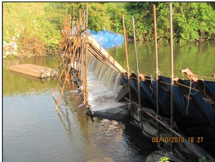
**Photo 4-13. Temporary Dam Structure in Reach 4**
