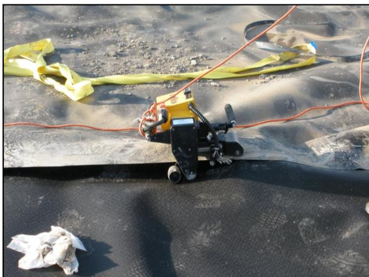
**Photo 4-4. Hot Dual Wedge Welding of LLDPE Liner Panels**
