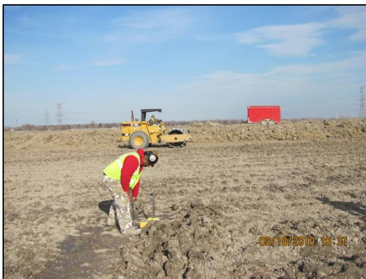
**Photo 3-1. Earthwork and Compaction Testing at Non-TSCA Dewatering Pad**
