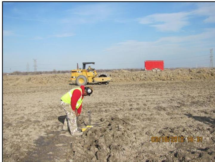
**Photo 3-1. Earthwork and Compaction Testing at Non-TSCA Dewatering Pad**
