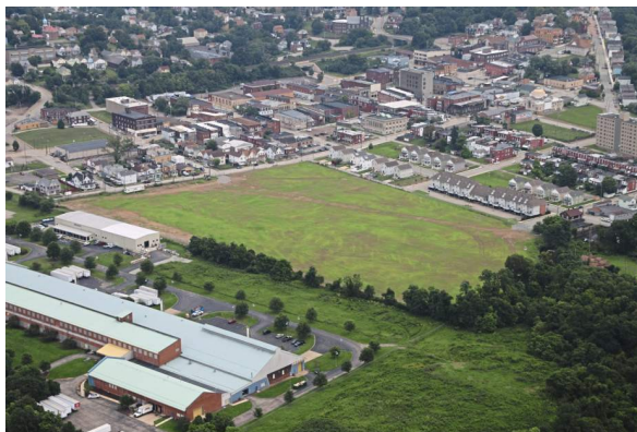
The 13.8 Acre Jeannette Glass Plant Site Preparation was Completed in Mid-2018
