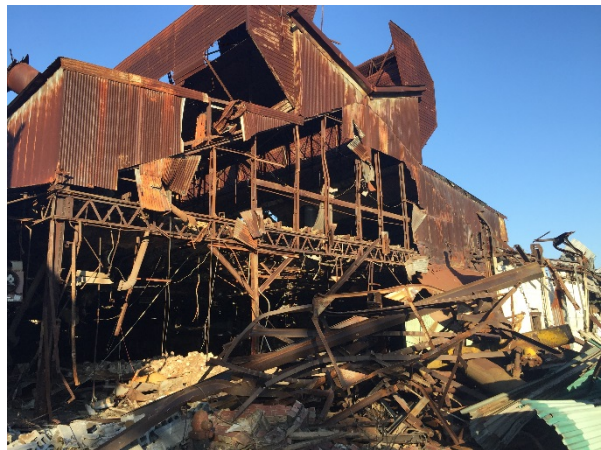
Former Jeannette Glass Plant Undergoing Demolition in 2017.
