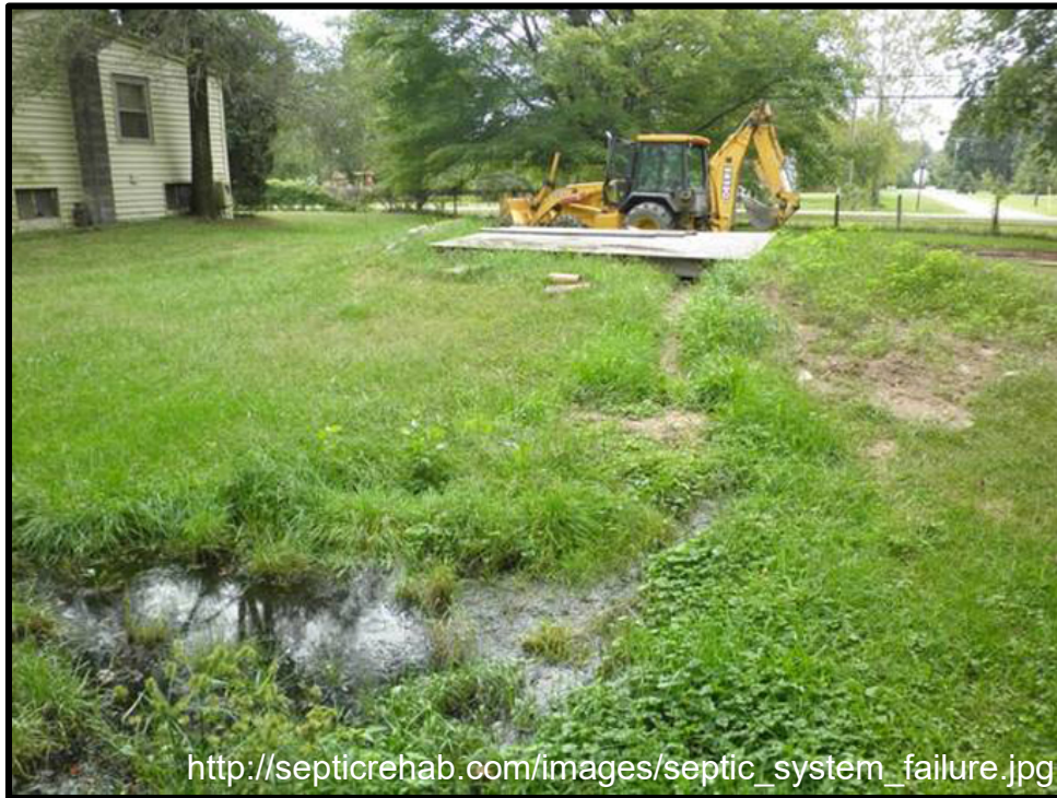
Failing septic system
