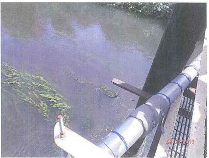
Description: The end of the intake tube for Monitoring Station 011 has weeds caught on it.
