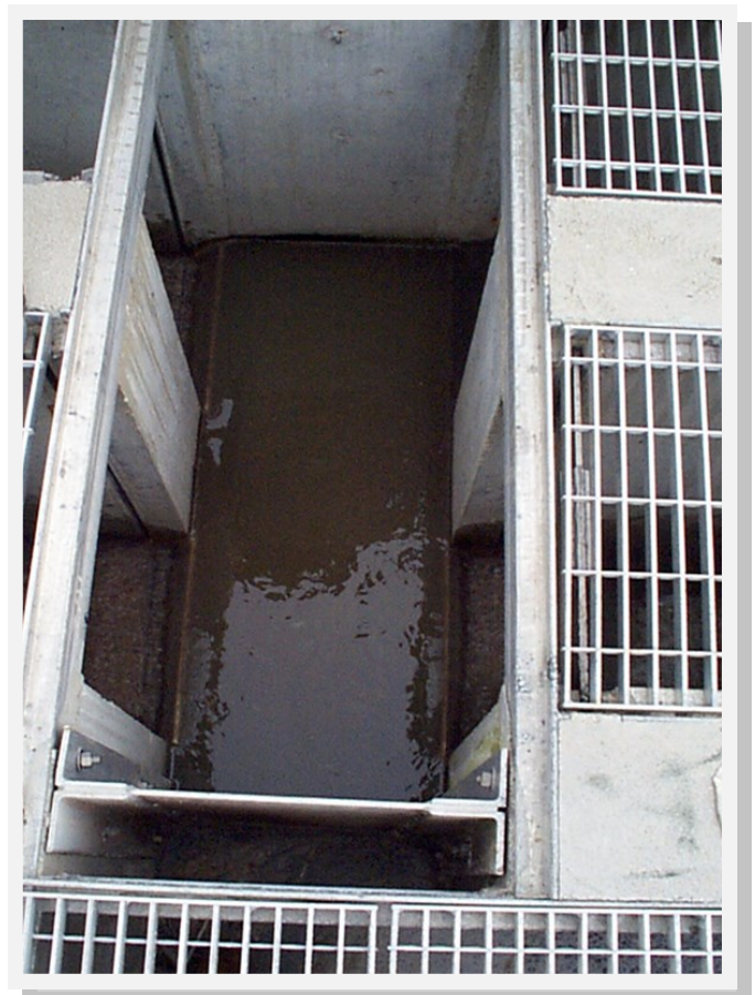
Proper Flow Splitter: Overflow weirs of equal length.
