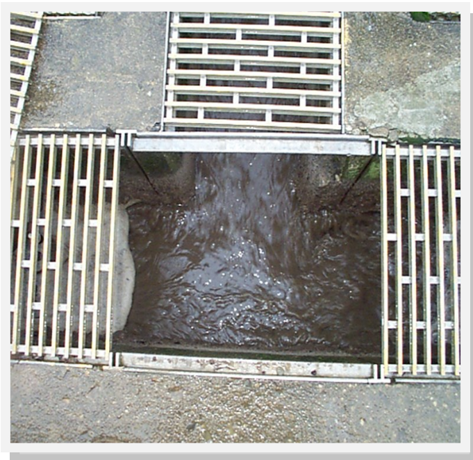
Random Flow Splitter: No weirs, no flow control.
