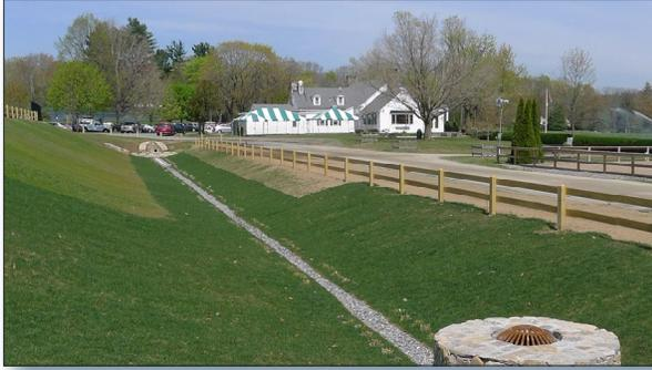
Figure 2. A stormwater runoff infiltration swale system was installed in 2012.
