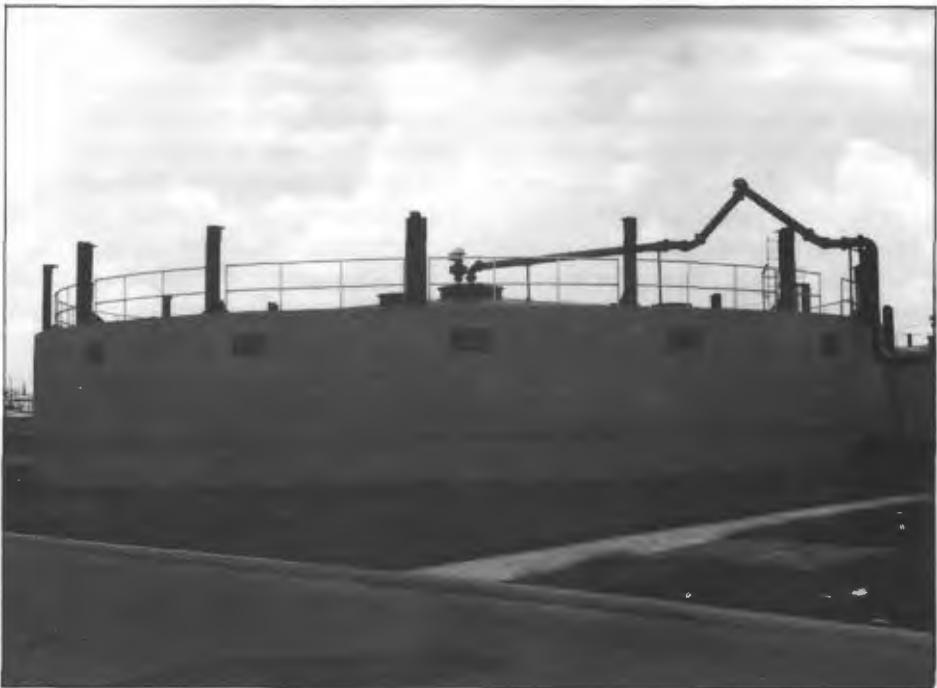
860,000-gallon anaerobic sludge digester with floating cover for storing the generated methane gas.
