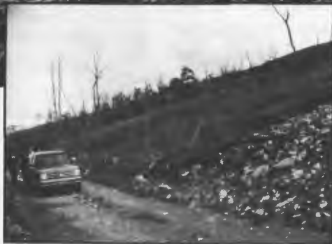
Above, truck spraying sludge/fly ash mixture for revegetation at the Palmerton, Pennsylvania hazardous waste site. Right, the same area after being reclaimed.
