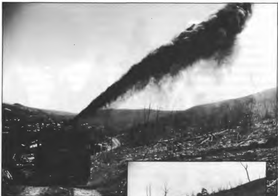
Above, truck spraying sludge/fly ash mixture for revegetation at the Palmerton, Pennsylvania hazardous waste site. Right, the same area after being reclaimed.
