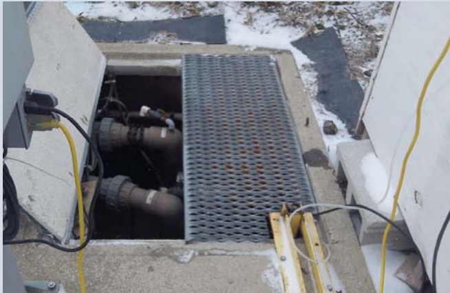
Flow Equalization Tank converted into Anoxic Tank
