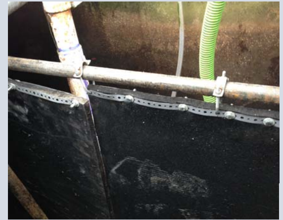
Aeration Tank Baffle Installed to Prevent Short Circuiting from Splitter Box to Clarifier
