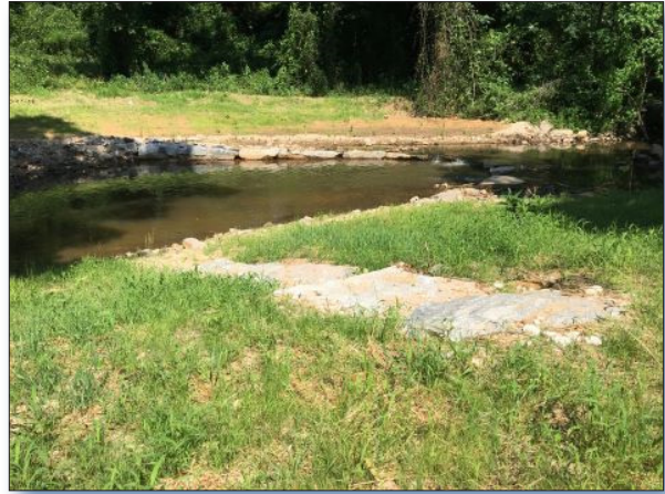
Figure 2. A boulder cross-vane redirects erosive flows.
