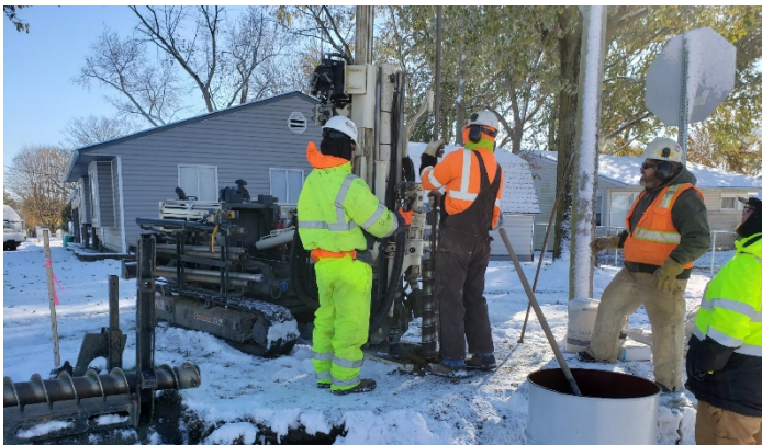
Photo #3: View of subcontractor installing monitoring well MW-36
