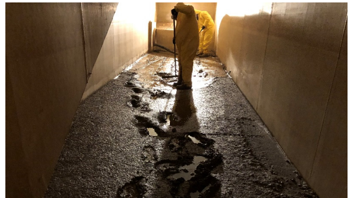
Photo #4: View inside the raw water tank during cleaning of sediment/sludge
