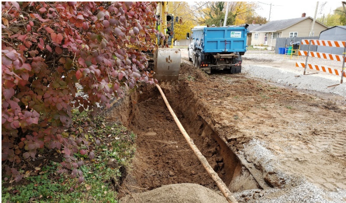
Photo #1: Excavation of former sewer line between MH #250052 and MH #250055, note the gas main
