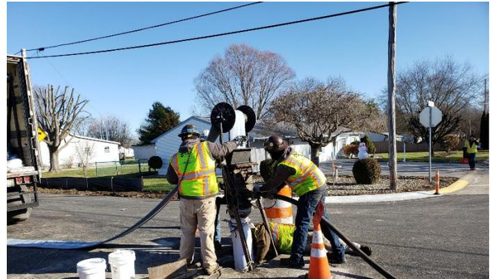
**Photo #4:** View of sewer lining installation from MH #250040 to MH #250010.
