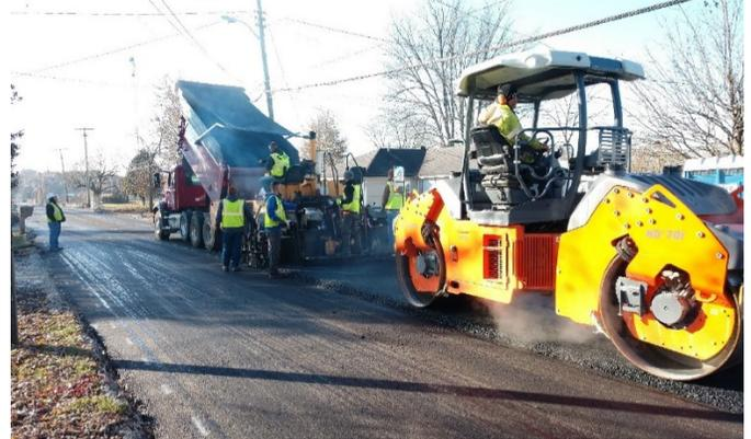
**Photo #2:** View during installation of the asphalt intermediate base coat for Forsythe Street
