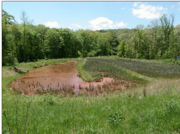
Figure 2. A settling pond and wetland were installed to address the BC16 AMD discharge site along an unnamed tributary to Blacks Creek.
