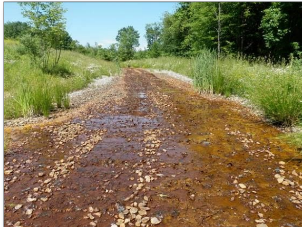
Figure 3. An oxidation precipitation channel (OPC) raises pH and removes iron from the water on a tributary that is downstream of the McIntire mine site.
