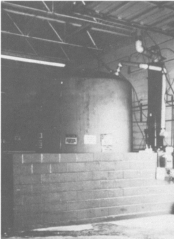
*A wall around an industrial storage container provides an effective control measure that prevents any accidentally spilled materials from entering the sewer.*
