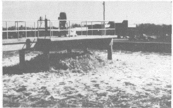
*Toxic industrial discharges can interfere with wastewater treatment by harming bacteria in biological treatment systems such as this aeration basin.*
