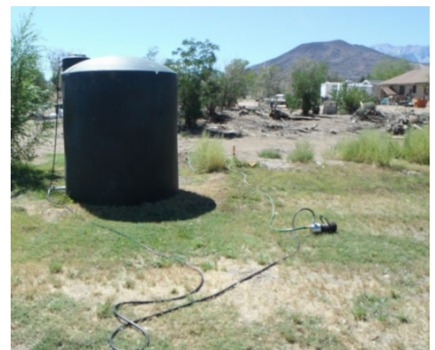
Figure 3. A residential irrigation system including a storage tank and small pump. Photo Credit: Alan Bacock, Water Program Coordinator.
