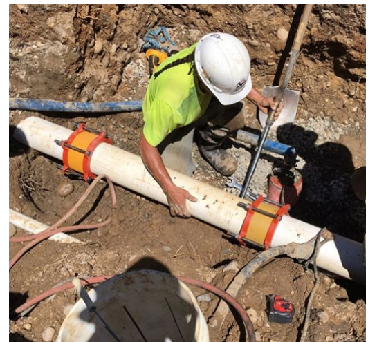
Figure 3. Torqueing the flange fitting to prevent future leaks. Photo Credit: David Weaver from Bishop Paiute Tribe
