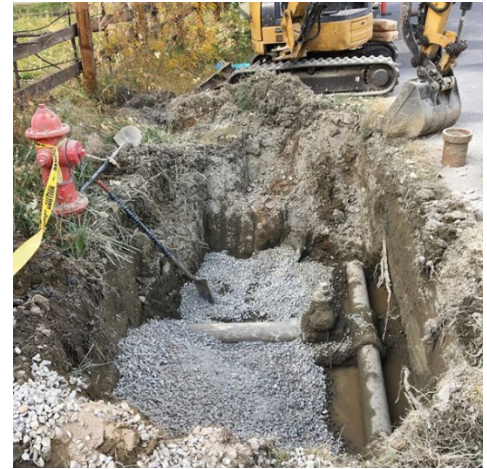
Figure 2. Replacing an old gate valve that had been leaking. Photo Credit: David Weaver from Bishop Paiute Tribe
