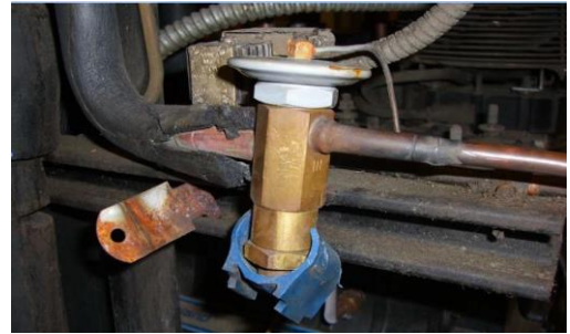
Image of broken clamp caused by vibrations
