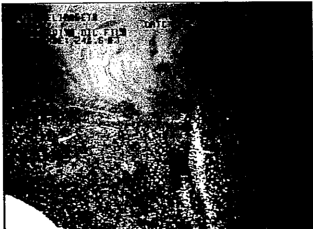
Photo: 65a, Tape No.: BM 2, 00:26:44 244.6FT, joint WITH OIL FILM
