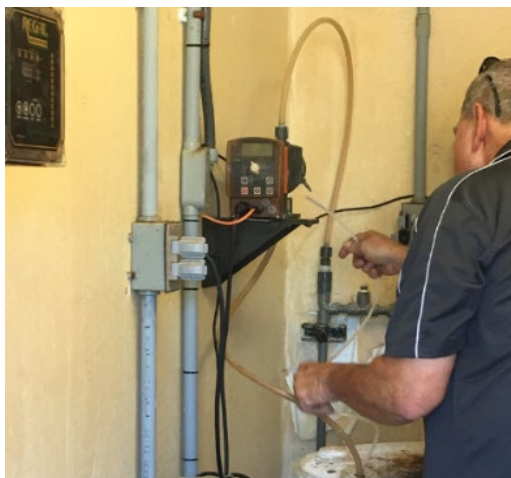
Figure 6. Checking calibration of chemical feed equipment. Photo Credit: PCIUA
