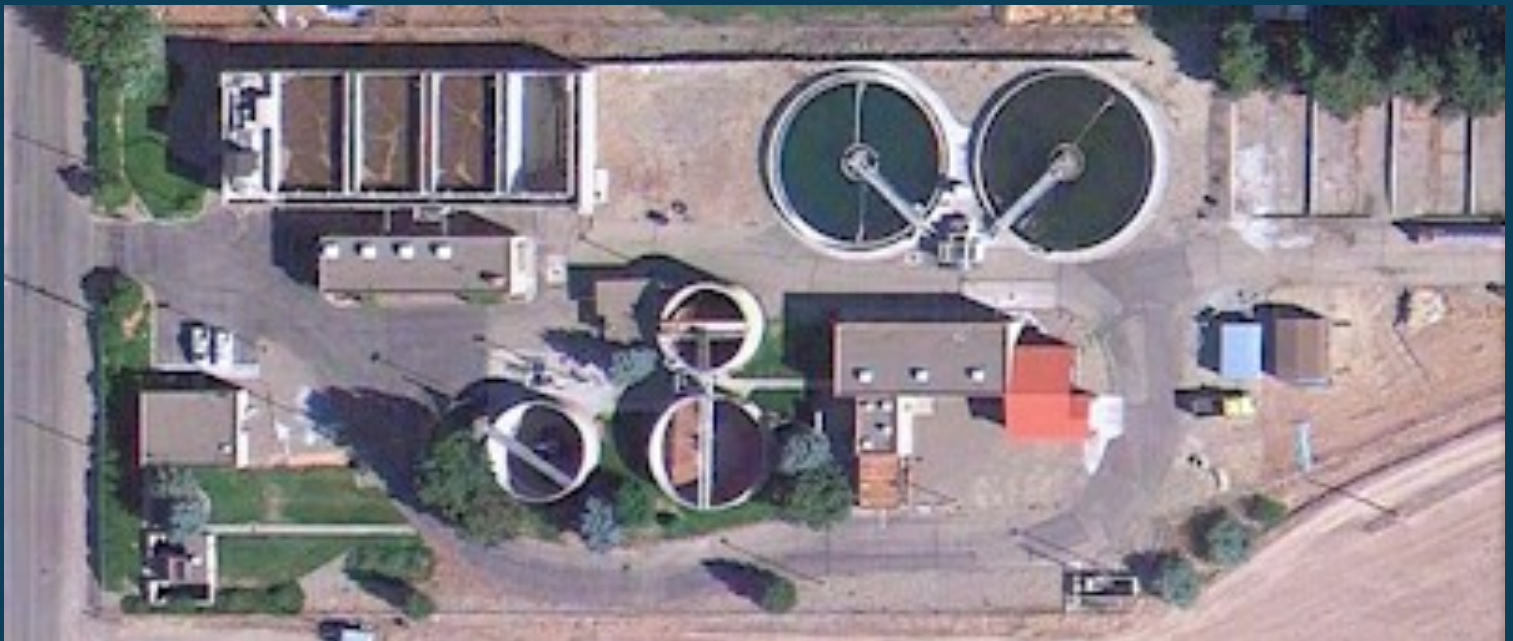
Bird's-eye view of City of Weiser WWTP
