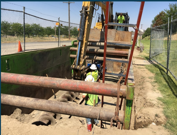
Crew doing directional drilling of new transmission main
