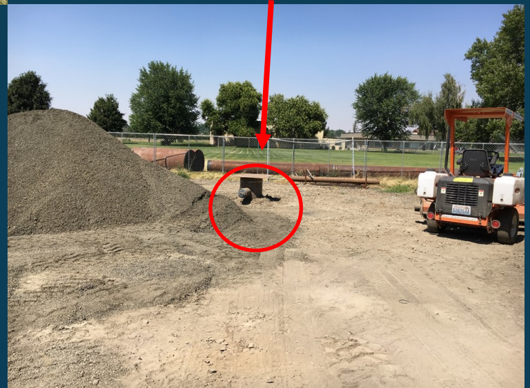
The new well
