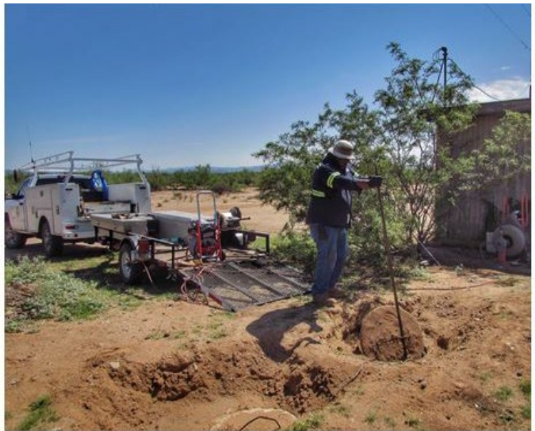
Figure 2. TOUA plumber accessing a sewer line. Photo credit: TOUA.
