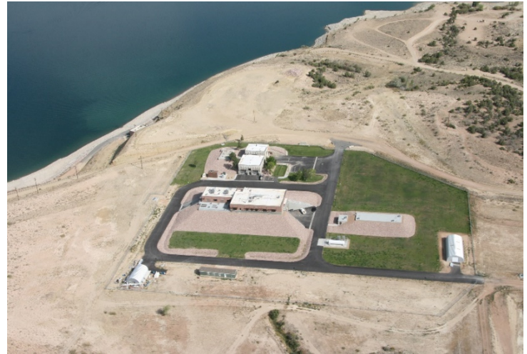
Figure 1. Duchesne Valley Water Treatment Plant
