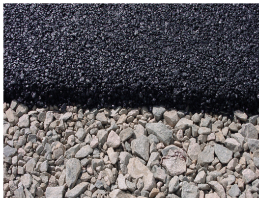
Porous pavement close-up, Aurora, CO. Courtesy of: The Colorado Association of Stormwater and Floodplain Managers (CASFM) .
