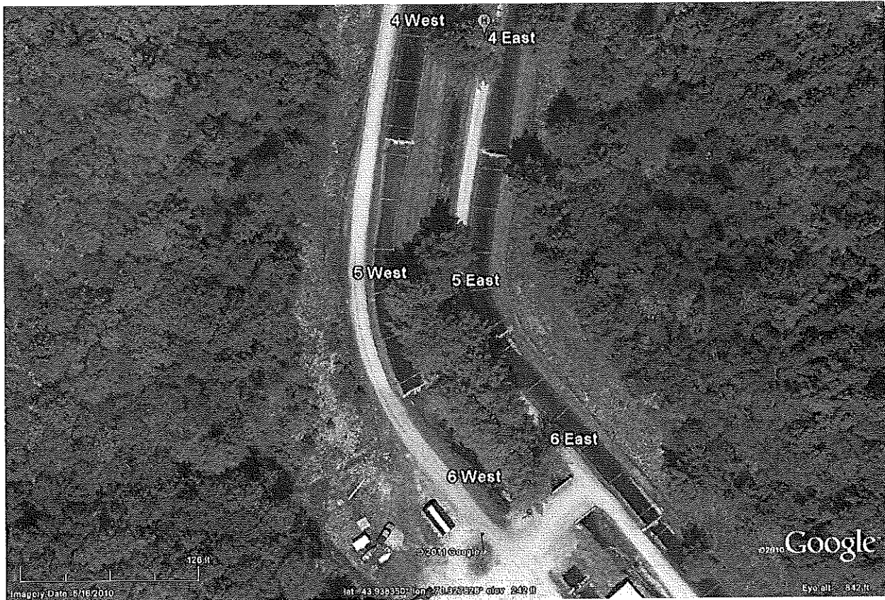
Figure 3 Raceways 4-6 West and East
