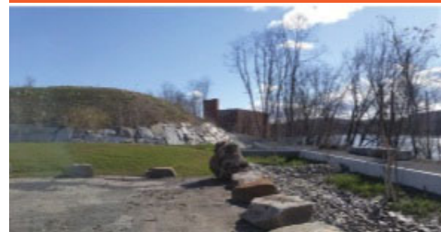
Figure 2 - Courtesy of the City of Lawrence, Mass.
