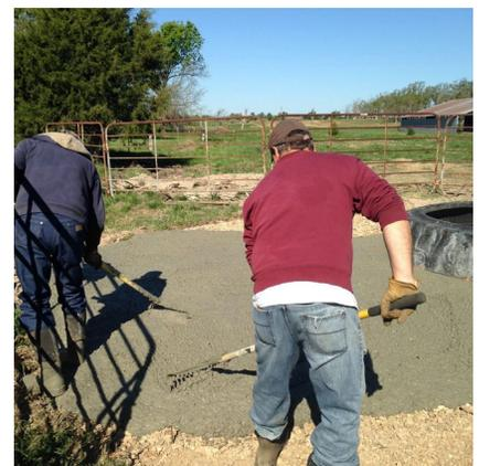
Landowners spread a concrete apron around an alternative watering tank.
