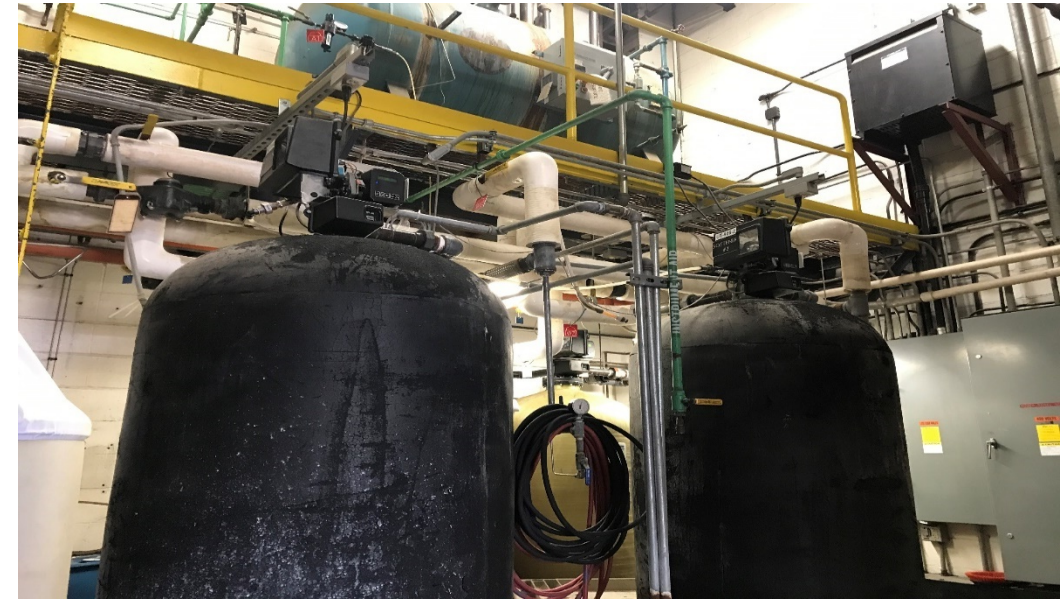
Water Softening for Boiler Water
