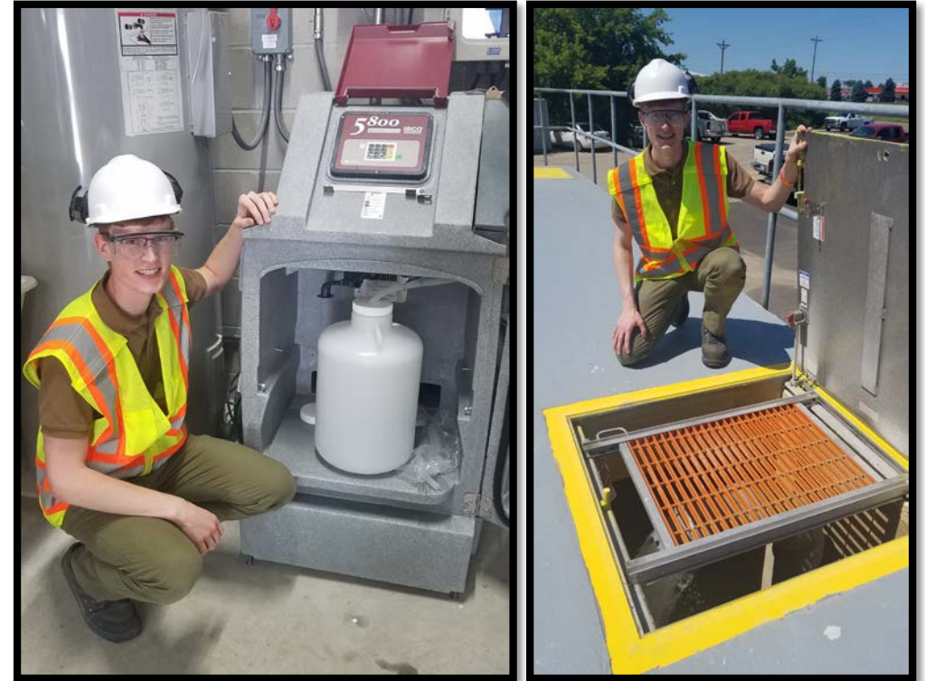
Figure: (L) Water sampler connected to waste system. (R) Access hatch to an adjustment tank
