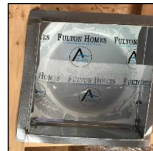
Example of customized duct covering from the 2018 Indoor airPLUS Builder of the Year Winner, Fulton Homes
