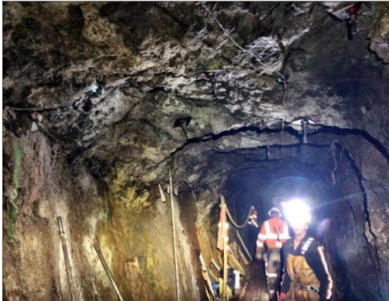
Stabilizing Bolts Reinforcing Rock Wall
