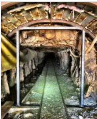
Better Drainage, New Rails
