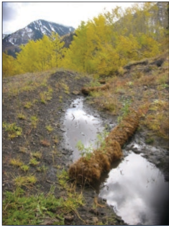
Figure 2. An erosion control BMP used to slow water flow along an old mining road.
