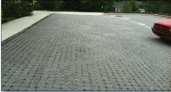
Figure 2. The town of Highlands installed permeable pavement at the Highlands Community Child Development Center.
