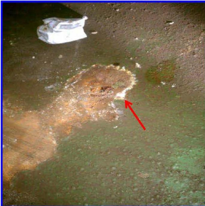
Visible salt on flat bottom of tank
