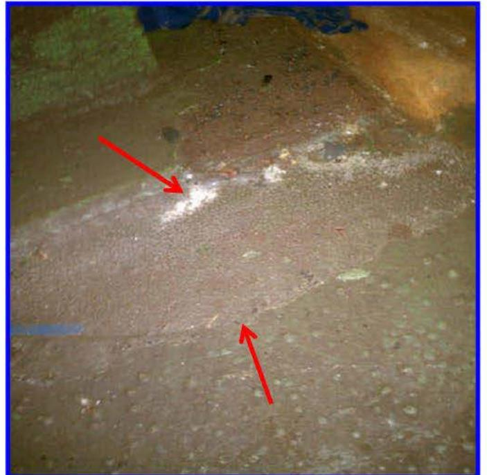
Visible salt on flat bottom of tank
