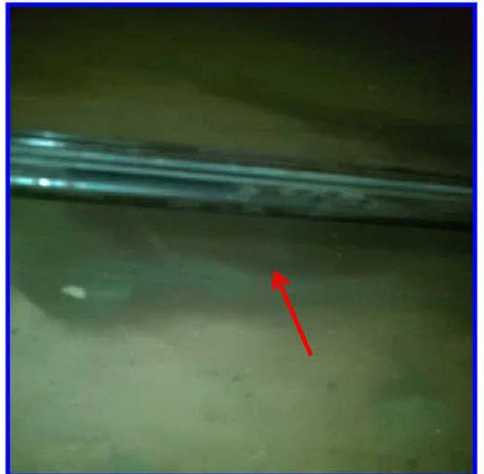
Visible grease under newly installed ppg
