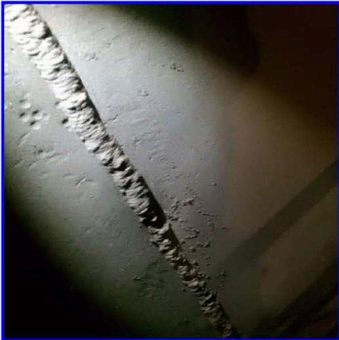
Length of weld with moderate to extensive weld spatter
