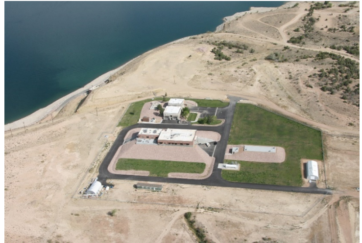
Figure 1. Duchesne Valley Water Treatment Plant
