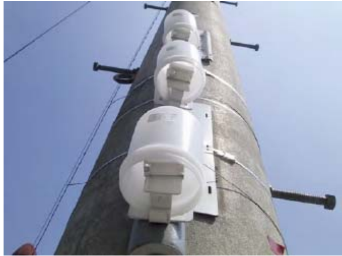
Figure 3. PSDs mounted on utility pole.
