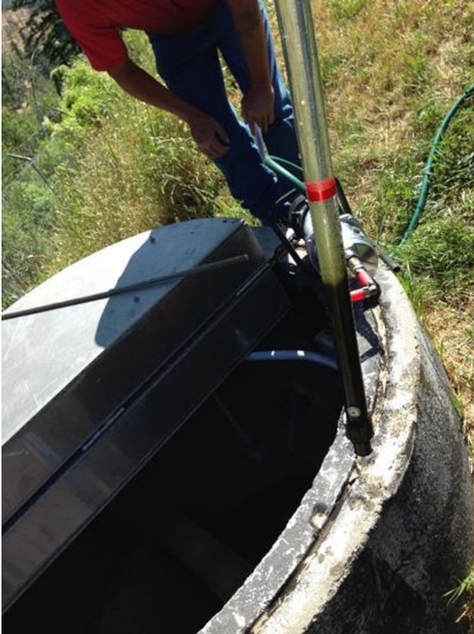
Sludge in the Discharge Well
