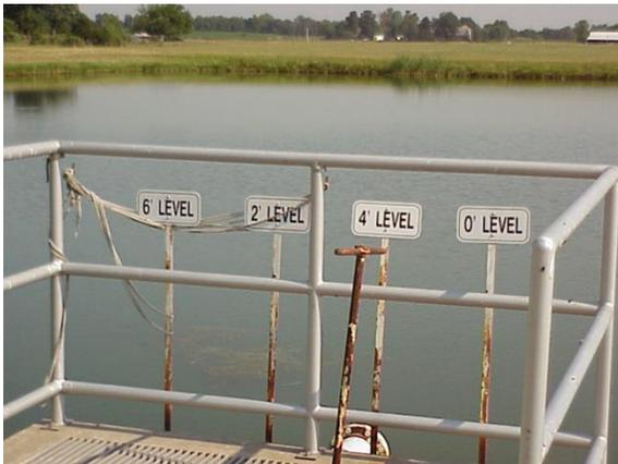
Because algae need sunlight, their concentrations are typically highest in the upper three (3) feet of a pond's surface. Pulling water from below this "photic zone" helps to minimize the discharge of algae cells.
