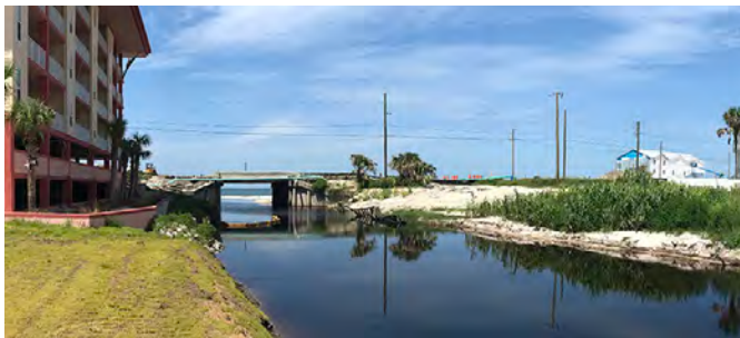
Existing 8th Street Canal opens to beachfront under Highway 98.
