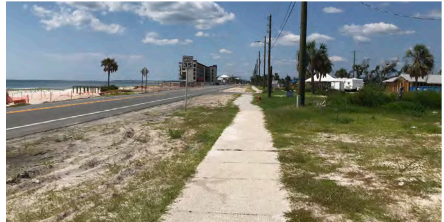
A wider multimodal sidewalk along Highway 98 and safe crossings to access the beach will increase safety for pedestrians and bicyclists.
