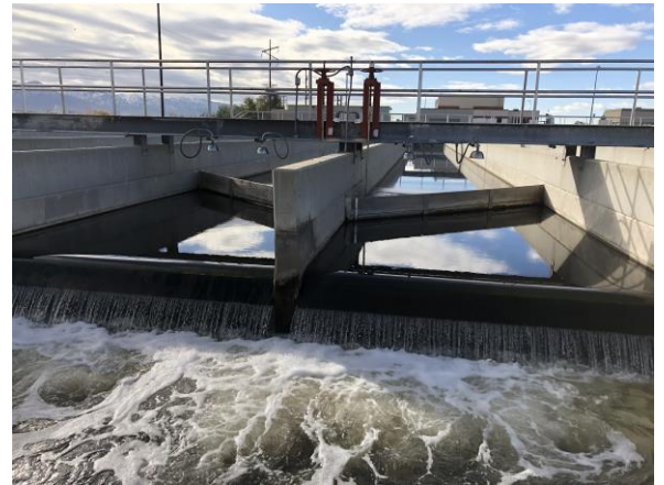
Water Reclamation Facility
