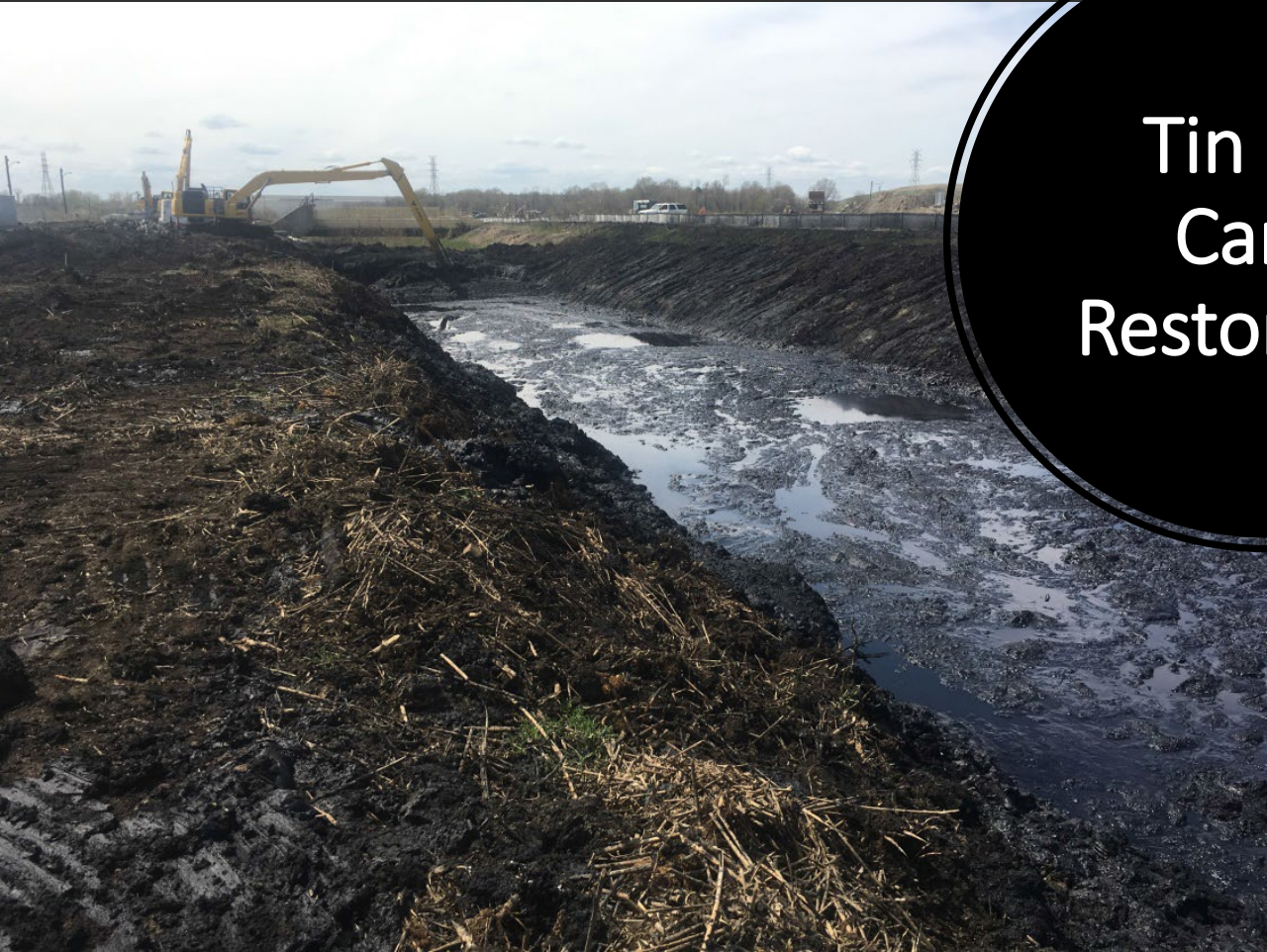
View of section #3 during sediment removal
