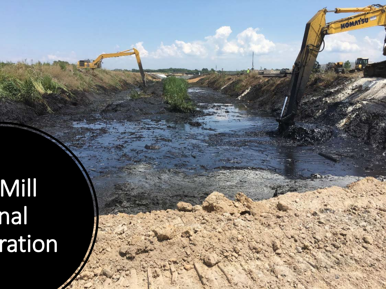
View of section #5 during sediment removal
