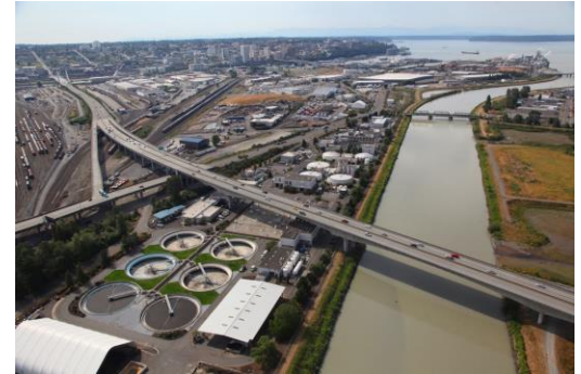
Central Wastewater Treatment Plant
