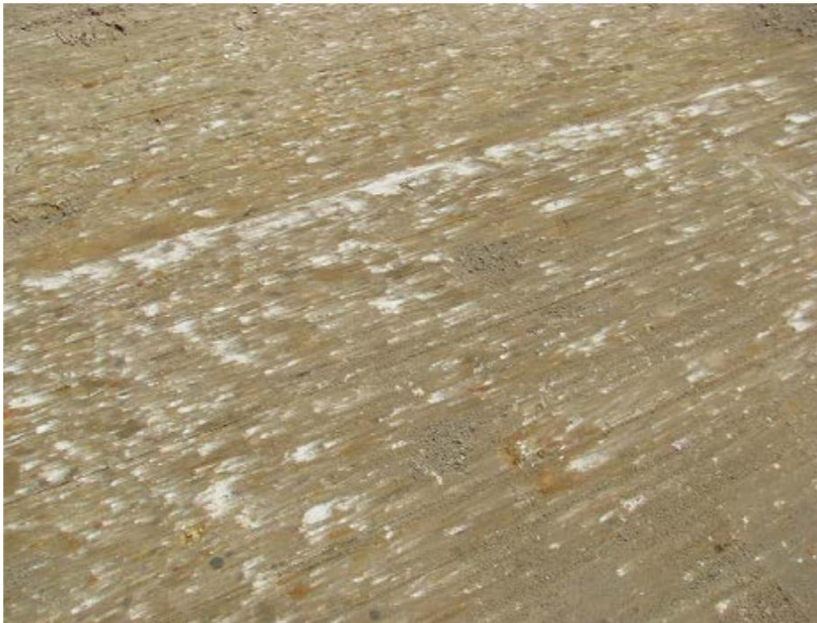
FIG. 49. Experimental road bed in Florida, USA, incorporating phosphogypsum (courtesy: Florida Industrial and Phosphate Research Institute).
