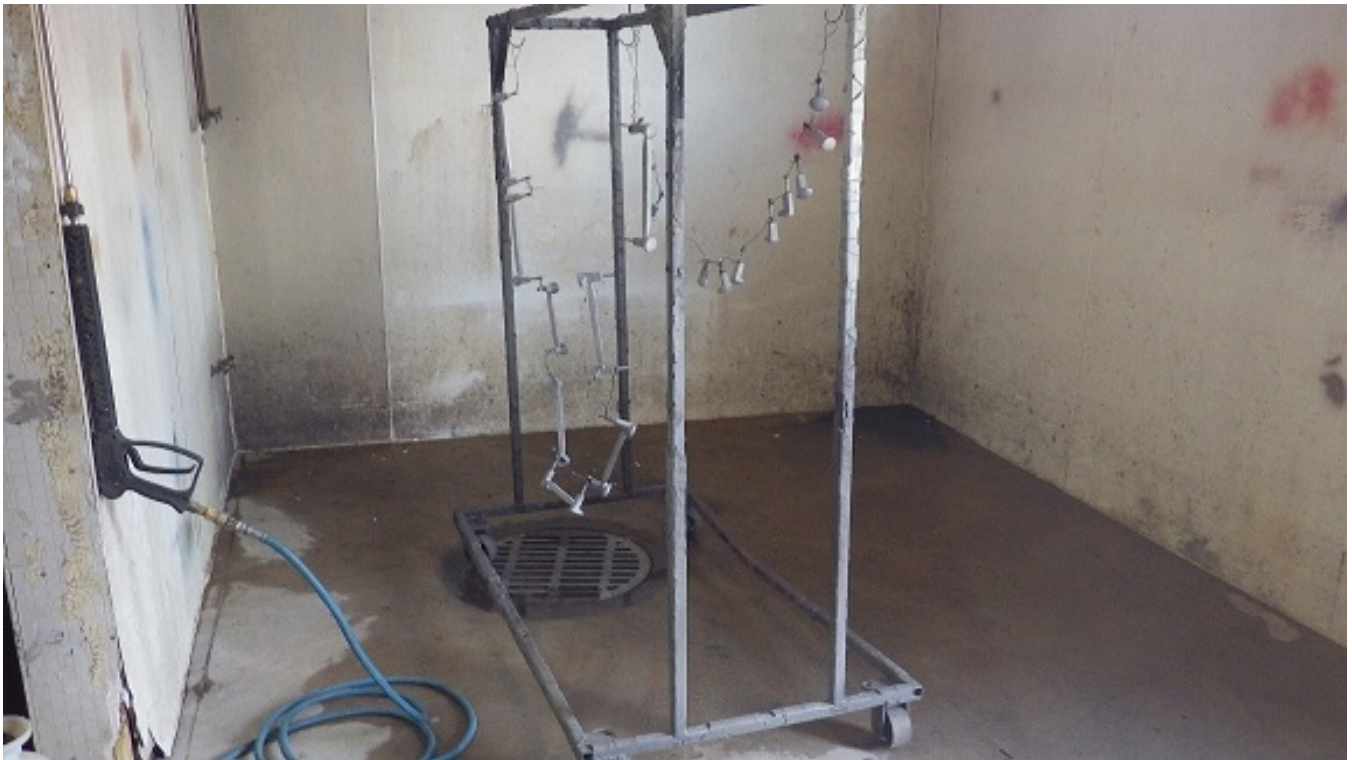
Figure 5 - Phosphate Spray Area
