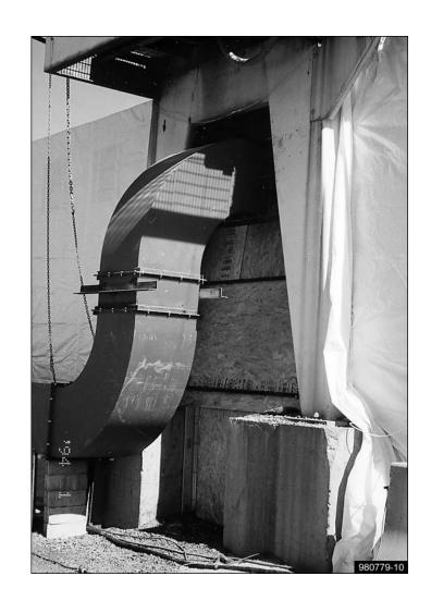
Figure 10. Close-up of Exhaust Duct Elbow (used for deposition wipe sample)
