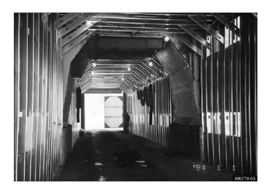
Figure 3. Empty Tunnel with Capture Hood/Loadout Chute in Center
