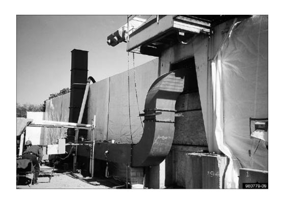
Figure 9. Exhaust Ducting, Sampling Ports, and Stack
