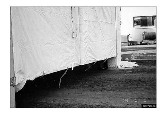
Figure 14. Makeup Airspace Along Doorway Bottom - Streamers Indicating Flow
