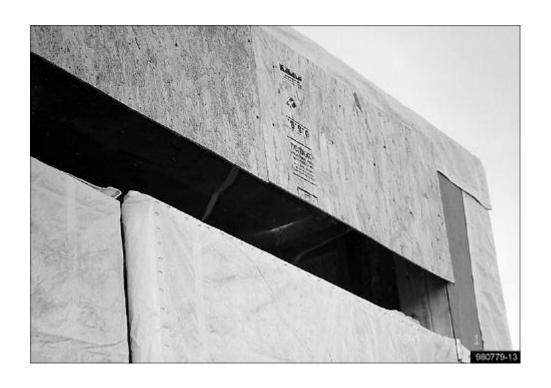
Figure 13. Makeup Airspace Along Doorway Top - Streamers Indicating Flow
