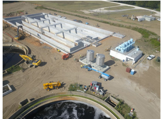
Disinfection Basin and Tank
