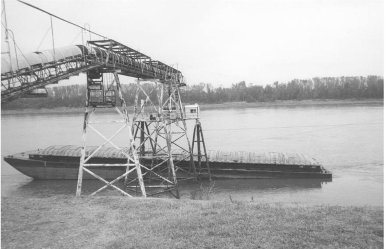
Photo 2. Continuous barge unloader.
