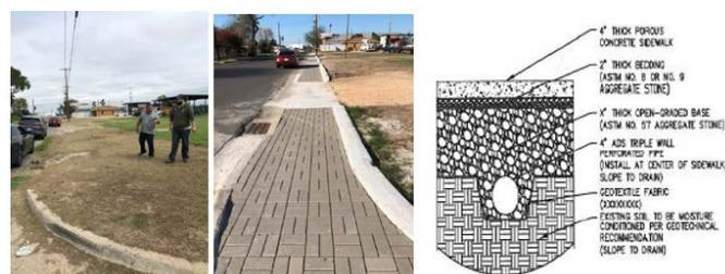
Figure 3. Before and after photos of high priority location, including engineer design of cross section of permeable pavement.
