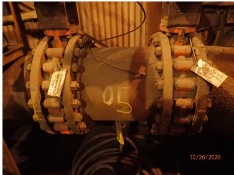
Description: Isolation Valves for Blast Furnace Recycle Sytem and Lake Water System on either side of an open empty portion of piping with a Bleed Valve below.
