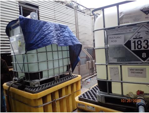
Description: Chemicals used to create chlorine dioxide are stored outside in totes. Chemicals are sodium chlorate and sulfuric acid.
