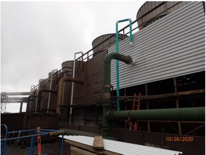
Description: Cooling Towers for the Blast Furnaces are being overhauled one at a time. The insides of the cooling towers have collapsed from the weight of the particles on the fill media inside. Location: Cyanide Destruct System.
