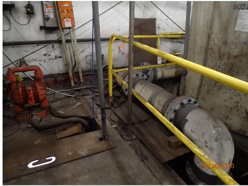
Description: White pipe is coming from the cooling tower outside the building that is being used to strip ammonia from the blowdown flow.
