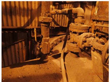
Description: Lake Water Intake pipe (through wall). Lake water flows at approximately 20,000 gpm through this pipe.
