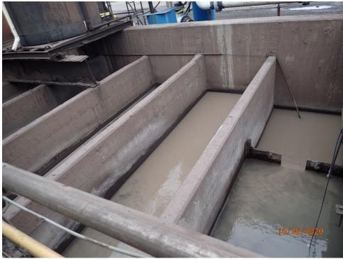
16: PA260016Description: Cell 4 of the Cyanide Destruct System. There is a a plume in the water that indicates a reaction of the chemicals in the water.Location: Cyanide Destruct System.Date/Time: October 26, 2020 11:46 A.M.
