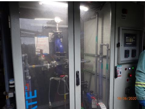
12: PA260012Description: Chlorine Dioxide Generator creates Chlorine Dioxide on site.Location: Cyanide Destruct System.Date/Time: October 26, 2020 11:36 A.M.
