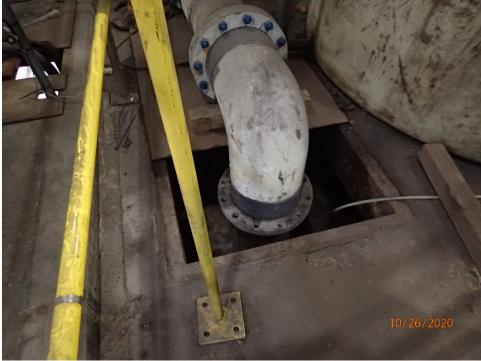
14: PA260014Description: Chlorine dioxide is fed into Cell 6 at the Cyanide Destruct System.Location: Cyanide Destruct System.Date/Time: October 26, 2020 11:42 A.M.
