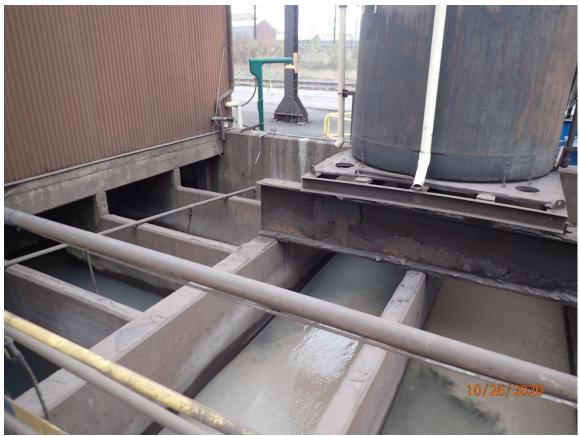
17: PA260017 Description: Cell 5 of the Cyanide Destruct System is on the left side of the photo and Cell 4 is on the right.
