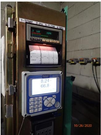
Description: Flow meter inside for Outfall 002 is inside the Sample Building. Flow on the meter was at 168,000 GPM.
