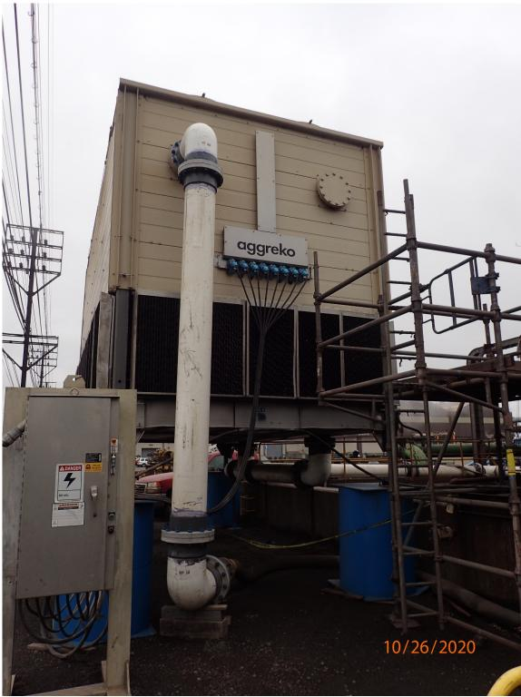
Description: pH of the Blast Furnace Blowdown is raised to 10 s.u. and then lifted to the top of the cooling tower for ammonia stripping. Cooling tower was rented and installed to investigate a way to reduce ammonia from the blowdown from the Blast Furnace Recycle System. Location: Cyanide Destruct System.
