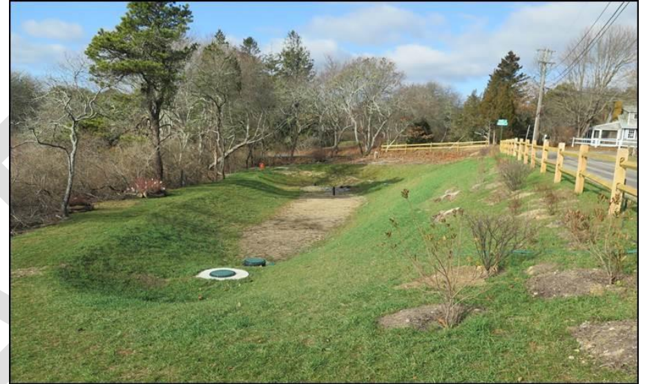
Demonstration of a Stormwater Gravel Wetland to Treat Runoff in Chatham, MA
