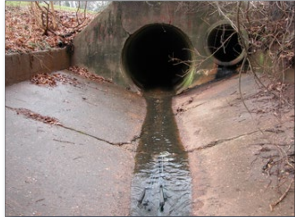
Figure 2. Before the restoration project, Candler Park Brook emerged from an underground culvert and flowed through a concrete channel.
