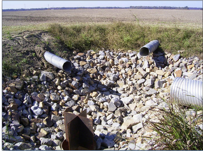
Figure 2. Four grade stabilization structures, including one antivortex structure.
